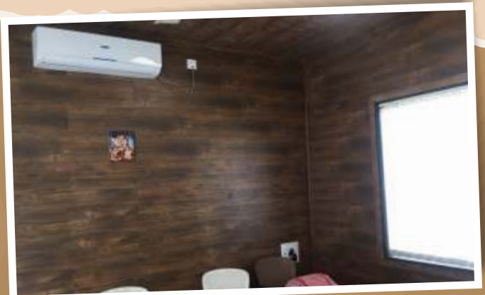
Cottage Velocity Project - Pune Flooring used in Wall Peneling
