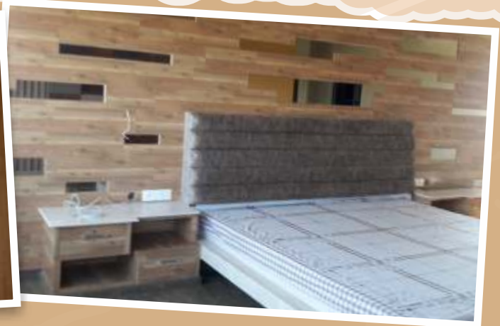
Flooring used in Wall Paneling in Hotel Room
